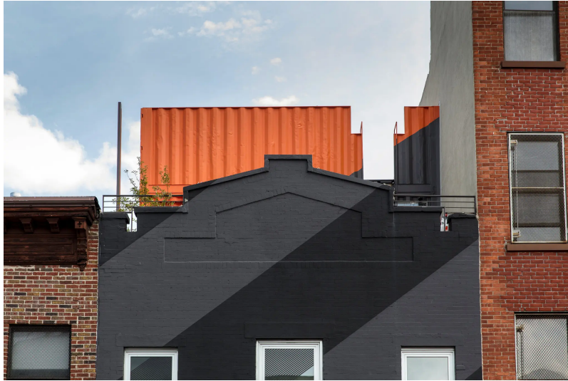
On Irving Place, in Clinton Hill, Brooklyn, a shipping container serves as a rooftop addition. Preston Schlebusch for The New York Times
